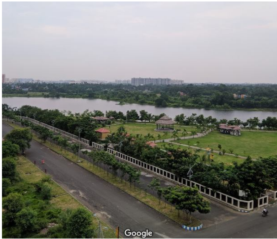
View showing existing boundary wall, pathways, lawns and thatched shelters
