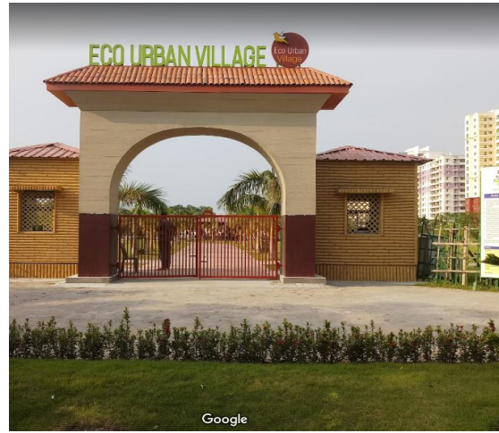
View of existing Entrance
